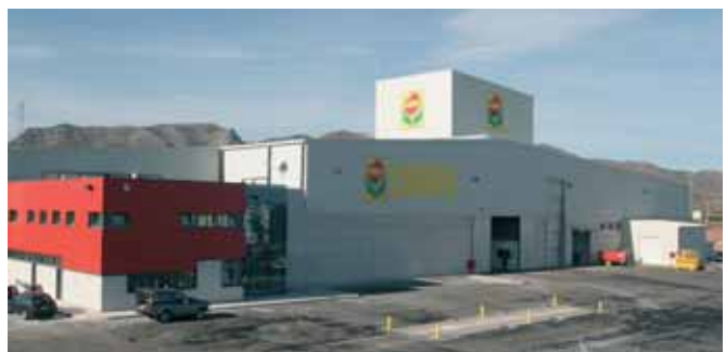
COMPO Vall d'Uixo production facility
